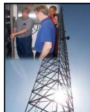
Public Safety Team: Ray Ryan, Radio Shop Manager for the City of Lincoln, shows the inside of the tower shelter to team members Mike Jeffres, Pam Kemper and Chris Heinze.
