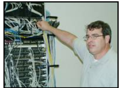
Mike Bittinger checking cables.
